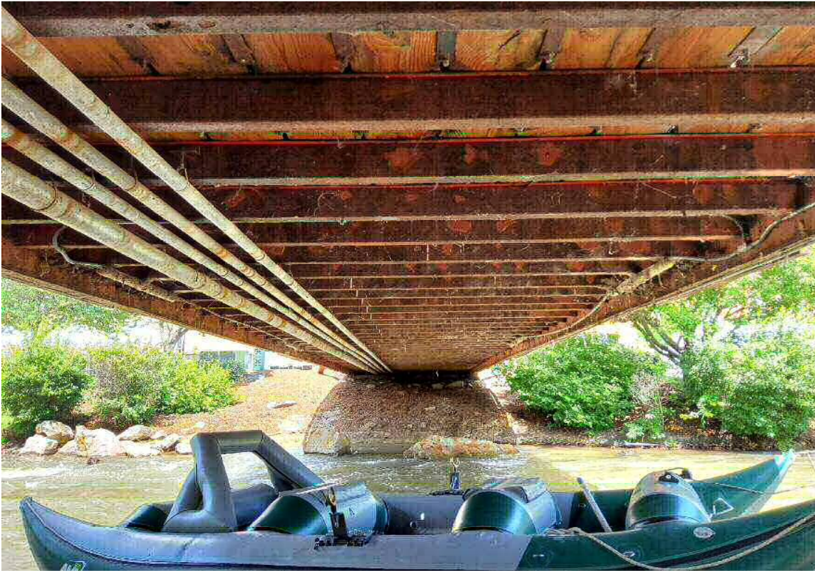
Description: Underside view looking North
