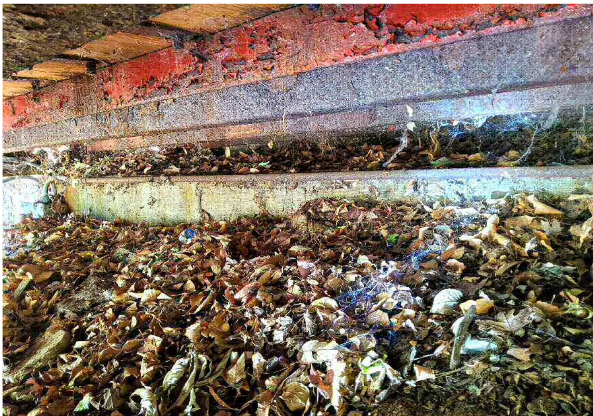
Description: Overall of south abutment
