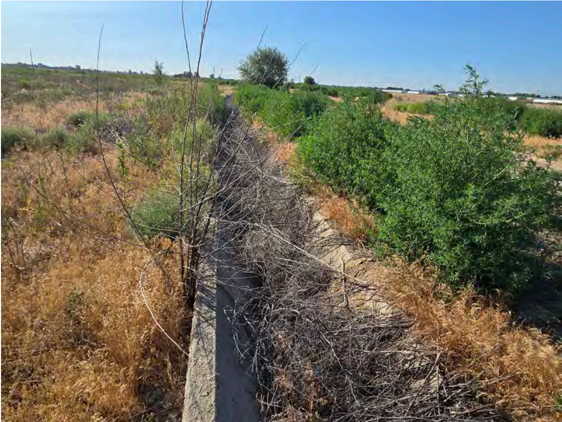
Figure 28: Portion of abandoned Canyon Hill Lateral within the Direct APE, facing southwest.
