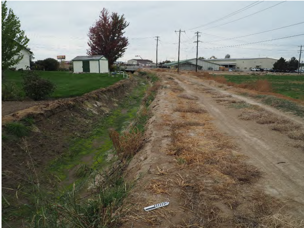
Figure 2. View of Canyon Hill Lateral (10CN111), facing northwest (10/13/2020)..
