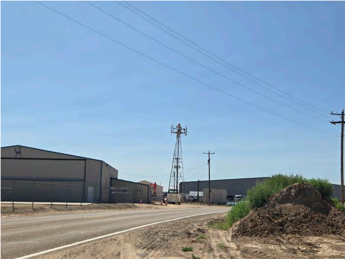
Figure 33: Example of existing infrastructure within the Caldwell Executive Airport, facing southeast.
