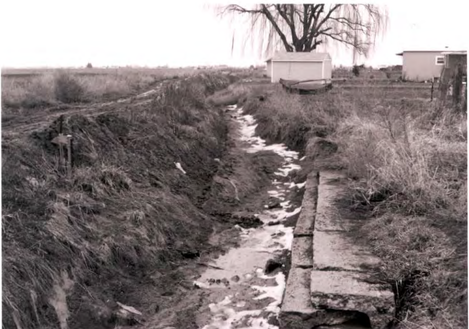
February 2, 2001 photograph of Canyon Hill Lateral to the southeast showing abutment and modern valve.
