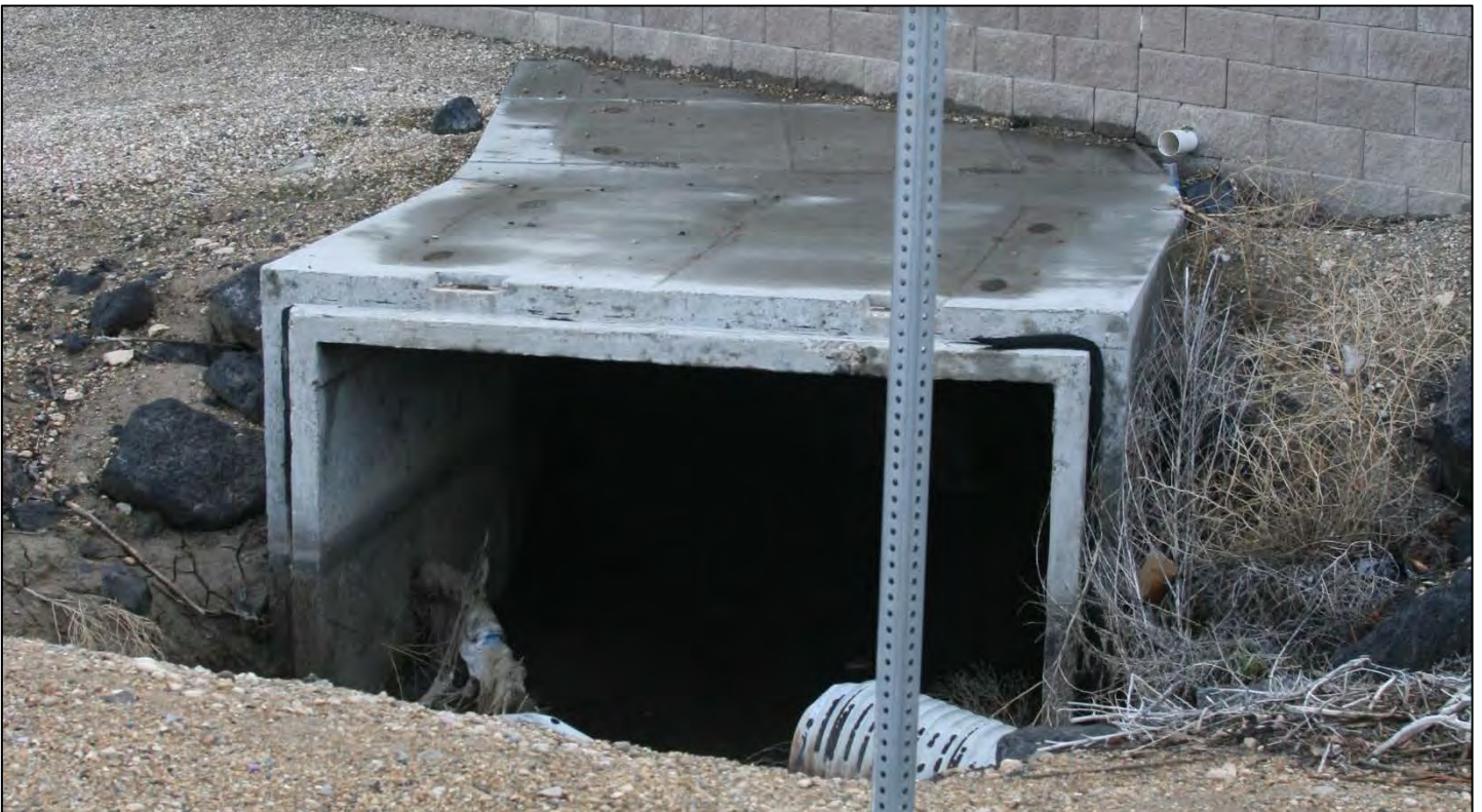
Canyon Hill Lateral as it exits the Franklin Interchange, camera facing south from Muller Dr.
