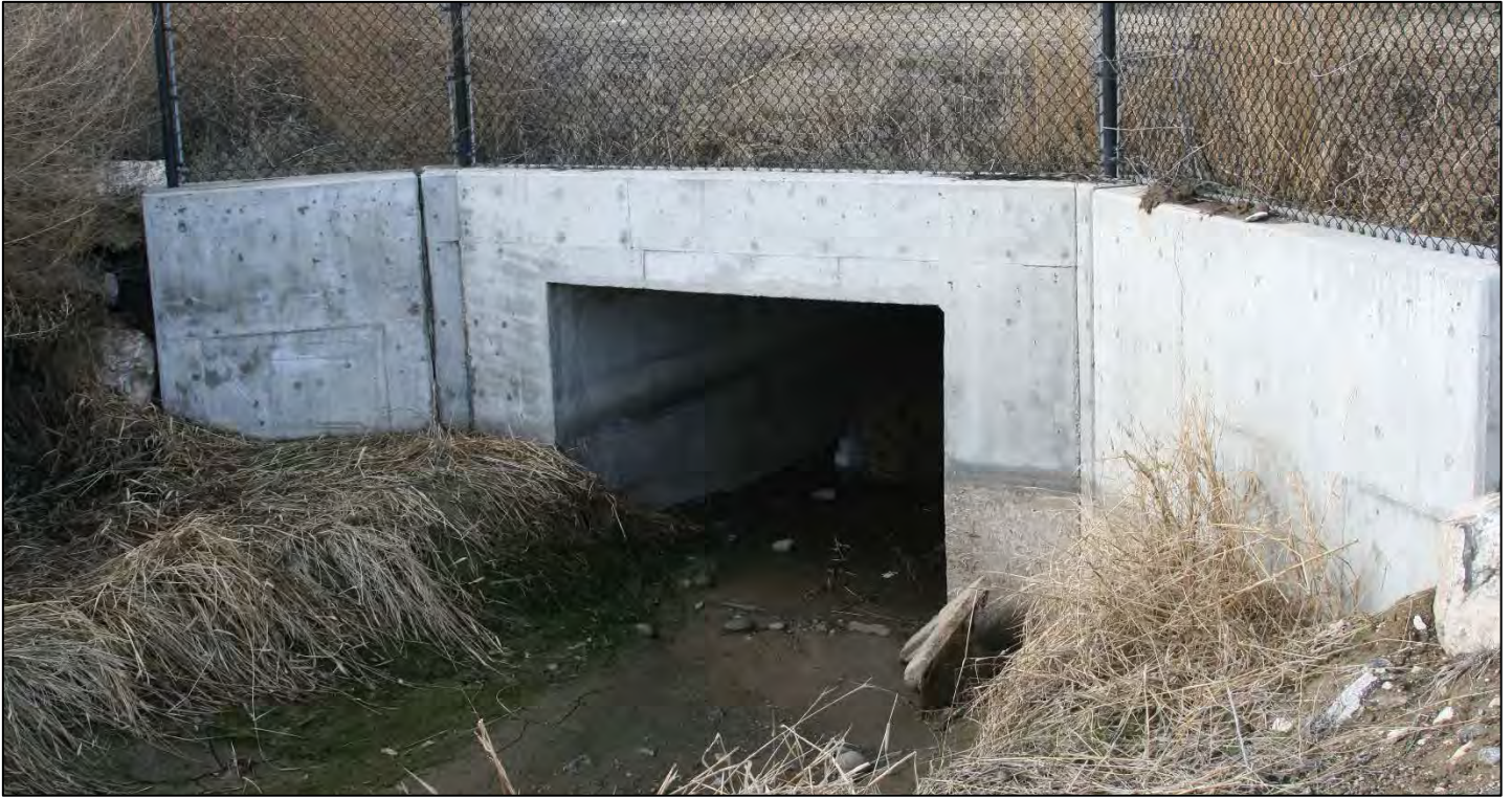
Canyon Hill Later culvert (approach) under the Franklin Interchange, camera facing northwest.
