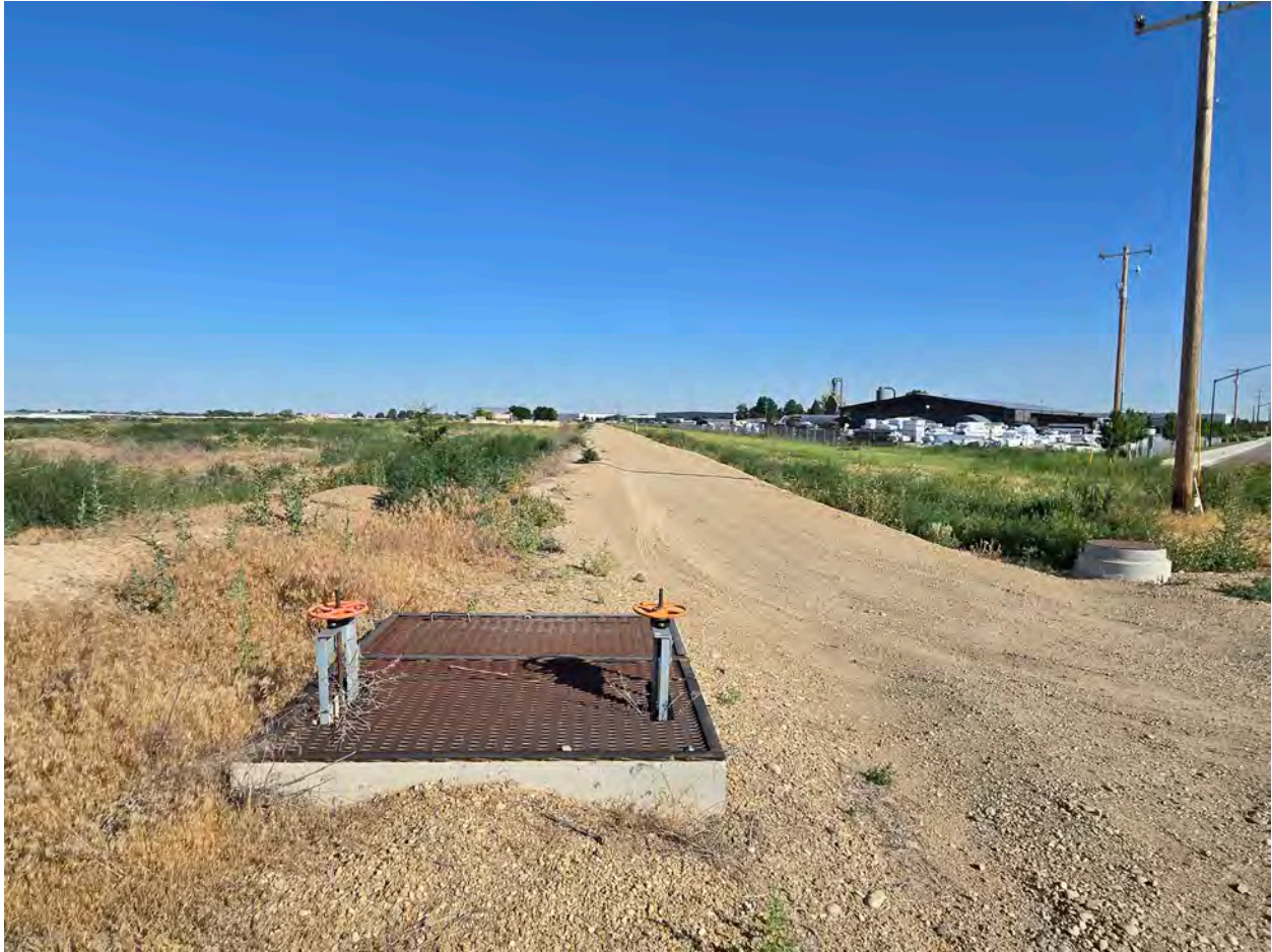
Figure 24: Existing infrastructure associated with piped Canyon Hill Lateral along South KCID Road, facing north.
