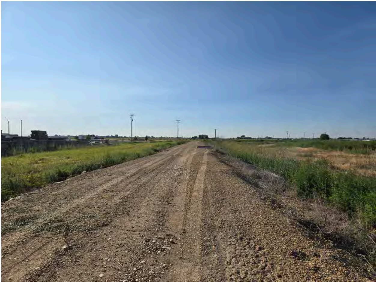
Figure 16: Overview of South KCID Road, view south.
