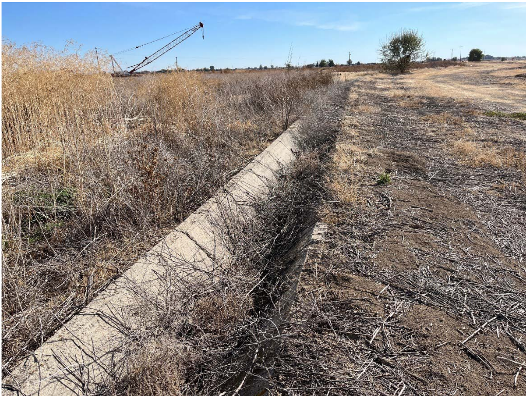
Photograph 2: East view of the abandoned relic Canyon Hill Lateral
