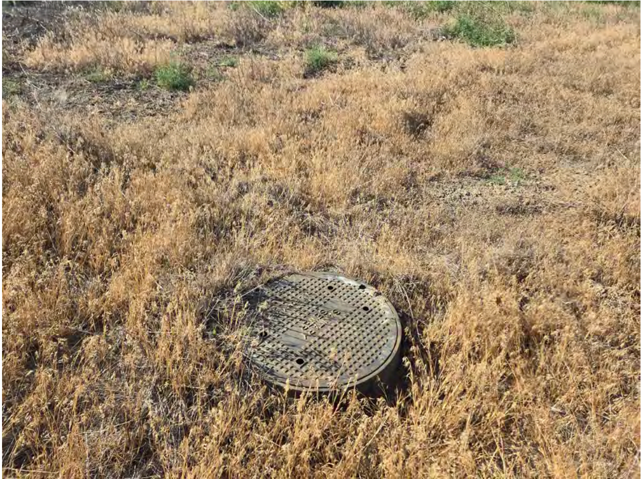
Figure 22: Overview of existing subsurface utilities, view down.
